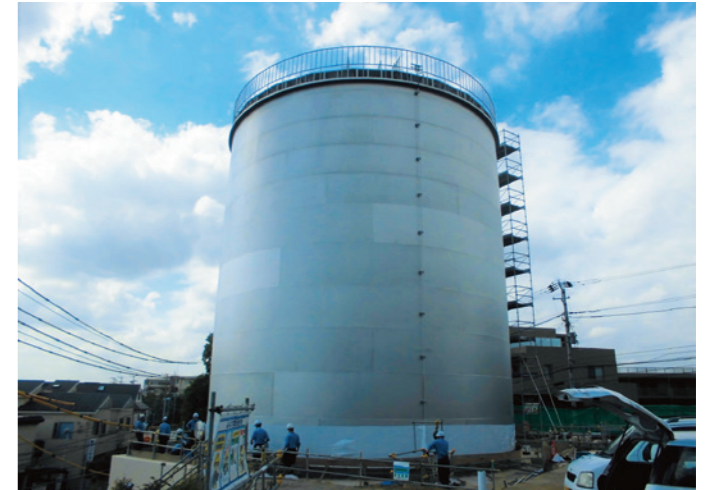
1,300m 3 配水塔 [13,500 φ ×14,800 H ]
